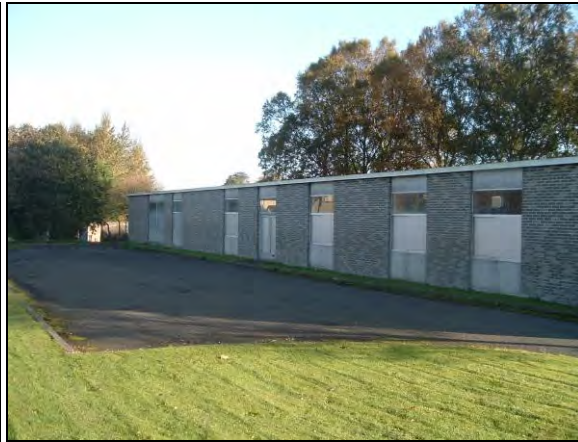
Plate 2 - West side of TSM building fronting onto Ard Easmuinn Road
