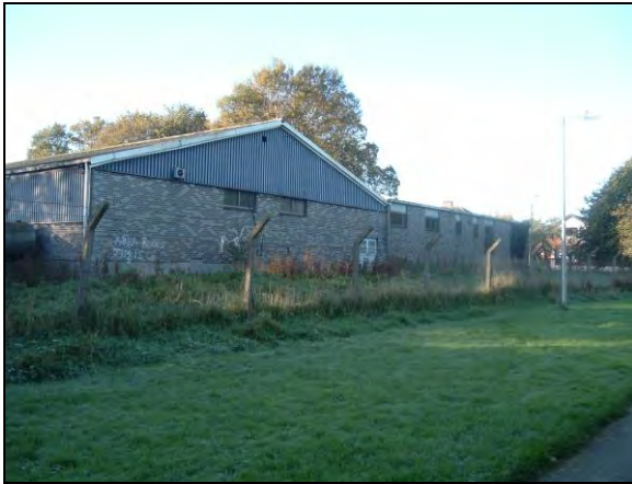
Plate 1 - North side of TSM building. Note dilapidated state of building
