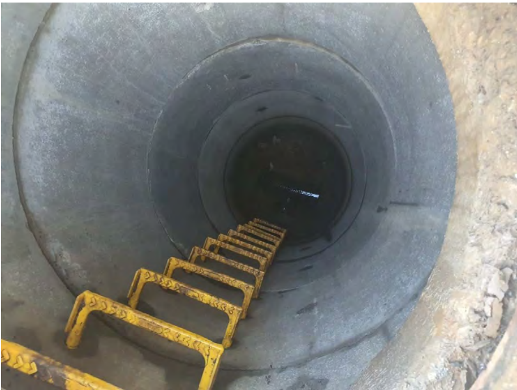
Photograph 5: Foul Drainage manhole at Location 2.
