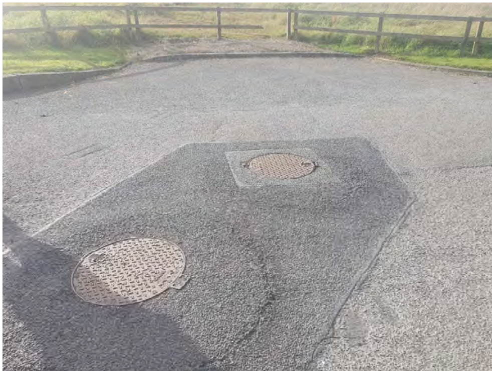
Photograph 3: Surface Water and Foul manholes at location 2 for connection.
