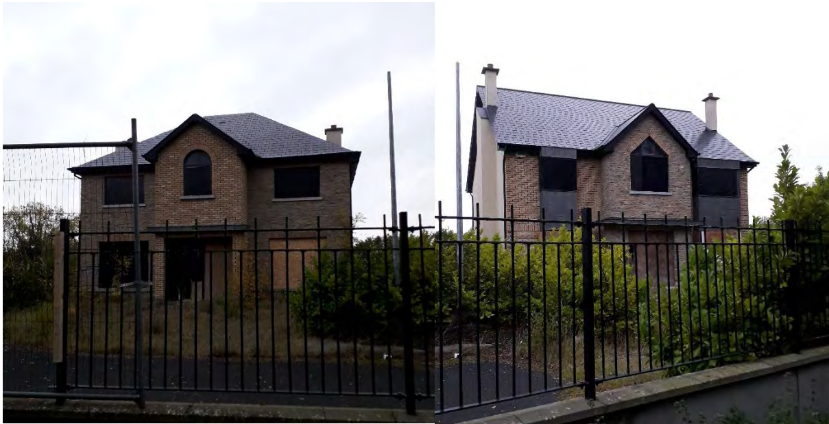
Figure 2: Two partially constructed two storey dwellings have now been completed and the balance of the development is well underway at Balfeddock Manor
