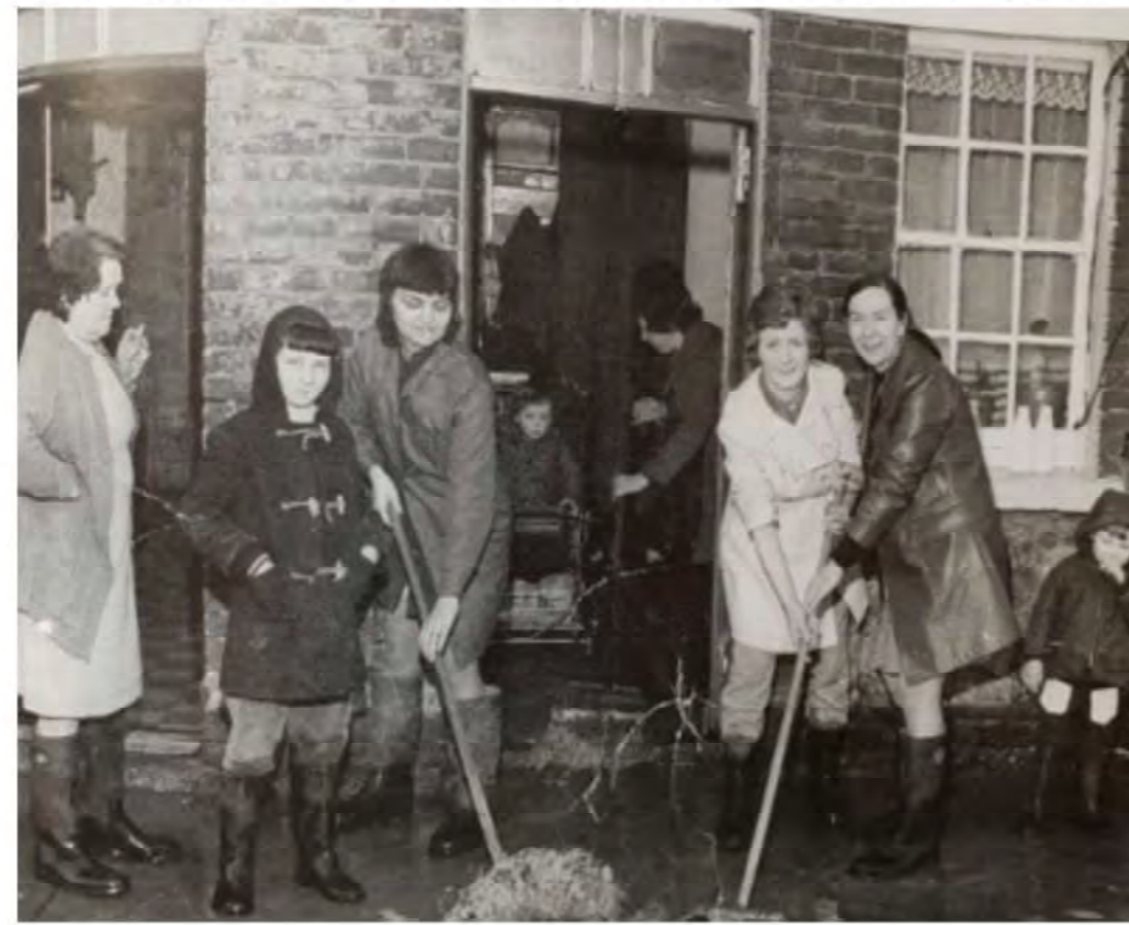
Plate 3.2 Images showing the original window configuration and door with glazed fanlight
