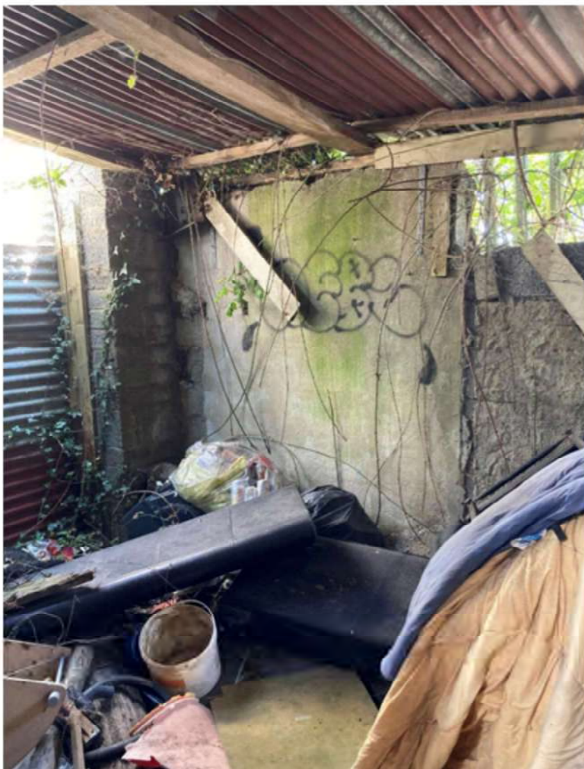
Plate 0.11 View within covered yard: Walls are constructed in a mix of stone, concrete block and corrugated metal cladding; a crude corrugated roof structure covers the yard.
