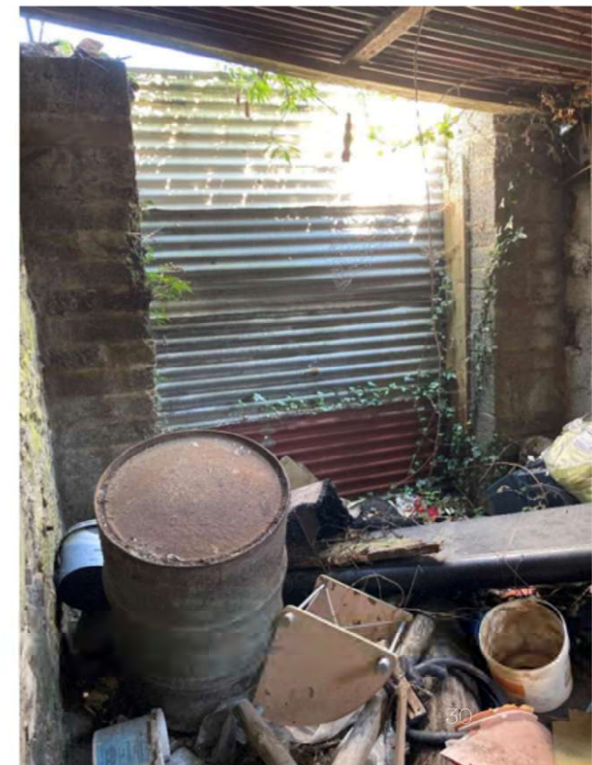
Plate 0.13 View of side entrance to rear yard.
