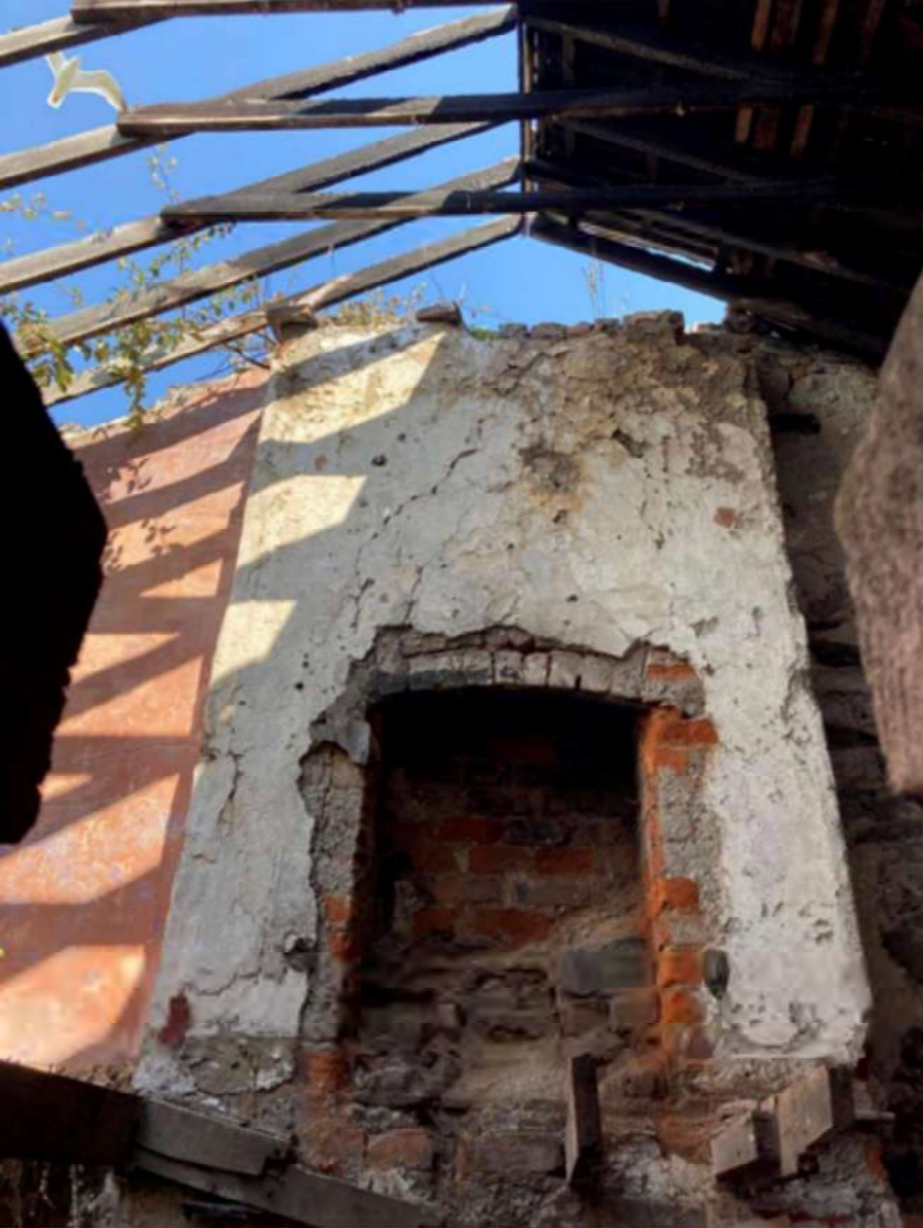
Plate 0.4 North wall showing: the chimney breast at upper level.
