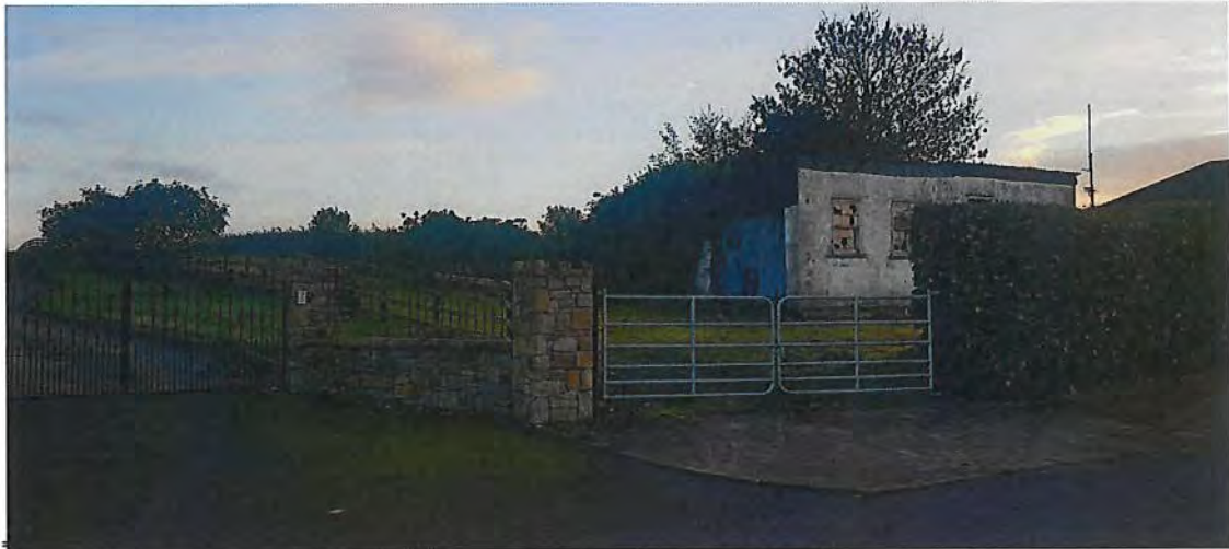
Photograph 1: Existing outbuilding on my land and existing entrance into the lands
