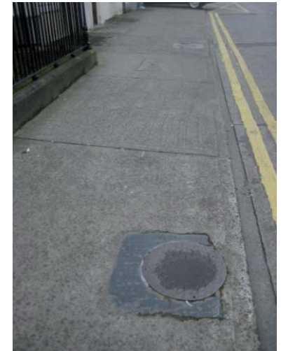
Figs 6.53 to 6.56: cast iron coal holes within pavements
