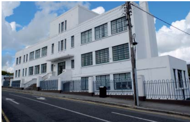
Fig. 6.36 Large scale mid-twentieth century building
