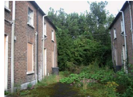
Fig. 6.23 Courtyard to St. John's
