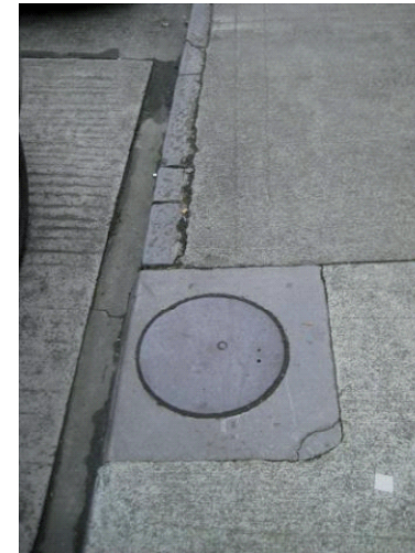
Figs 6.53 to 6.56: cast iron coal holes within pavements
