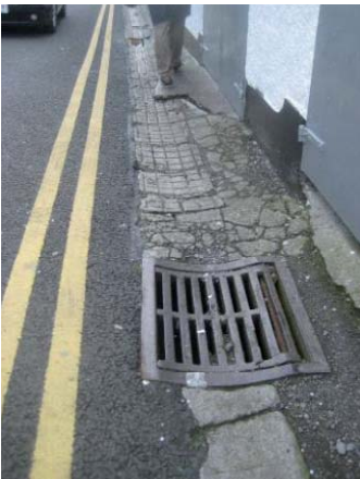
Fig. 5. 22 Fairgreen: Cobble drain and iron gully
