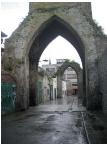
6.41: 'Abbey Lane': A most distinctive and unusual element of Drogheda's public realm is the lane which has been formed out of the ruinous Abbey church, running east-west through the former chancel and nave. This idiosyncratic feature deserves to be better presented, maintained and integrated. The architectural and archaeological significance of the monument needs to be preserved within the context of improved urban integration and information should be provided
