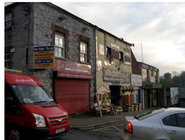
Fig. 5. 15. West Gate: A section of upstanding medieval wall survives behind a temporary hoarding and the spatial character of this place reflects its historic gateway origins. However, the potential of this space is compromised by its surface car park use, fragmented built edge and dominance of passing traffic.
