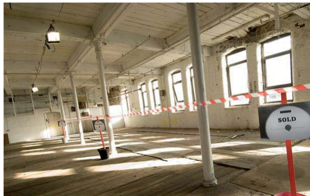
Fig. 6.31 Albert Mill, Manchester, interior before conversion (source: Urban Splash)
