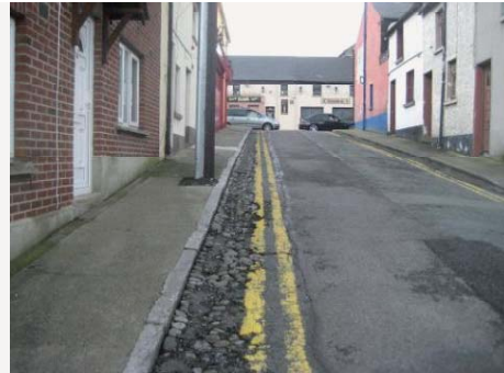
Fig. 5. 20 Limestone kerbing and cobble drain
