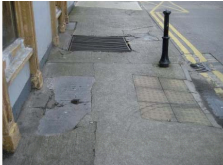
Fig. 5.19 Surviving limestone flag and pavement grille within modern pavement.
