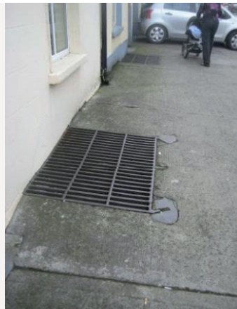
Fig. 5. 23 iron pavement grille, basement area, Fair St
