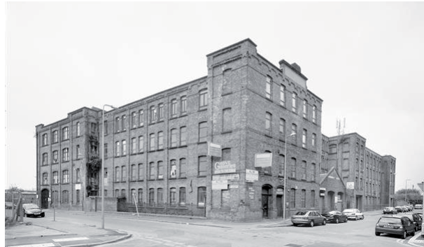
Fig. 6.29 Albert Mill, Manchester, before conversion (source: Urban Splash)
