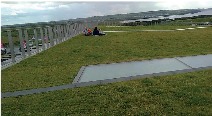
Fig. 6.94: Green Roof/public space - Giant's Causeway Centre
