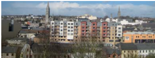
Fig. 6.37 Recent large scale building onto River Boyne.
