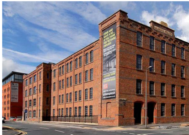
Fig. 6.30 Albert Mill, Manchester, after conversion (source: Urban Splash)
