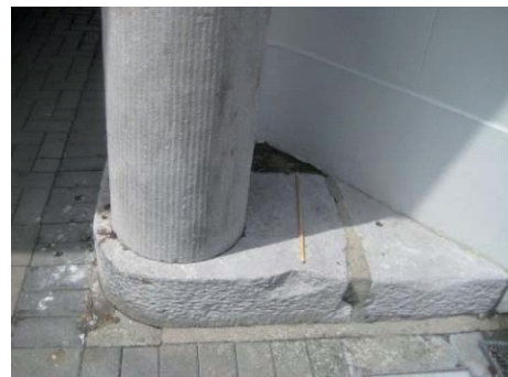
Fig. 5. 27 Limestone base to pillar at Drogheda Borough Offices entrance
