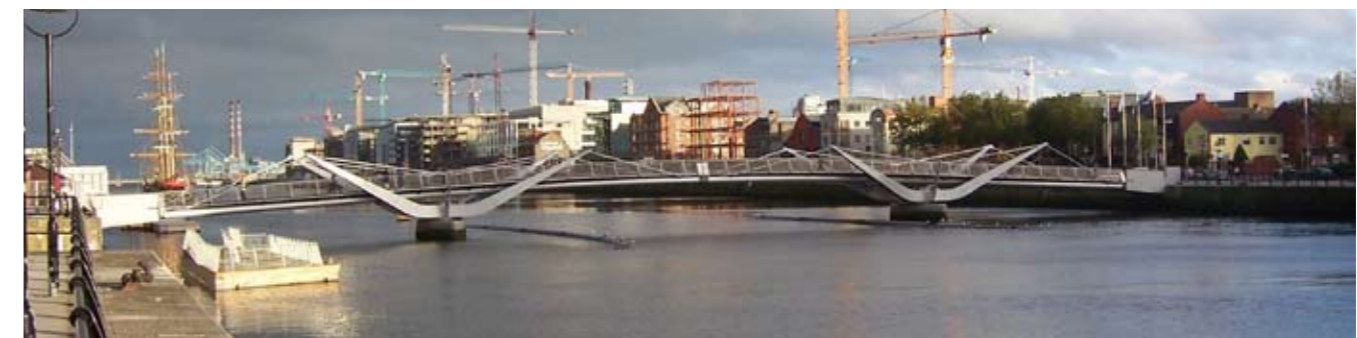
Opening pedestrian bridge
