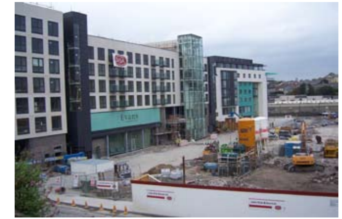
Scotch Hall development at Marsh Road
