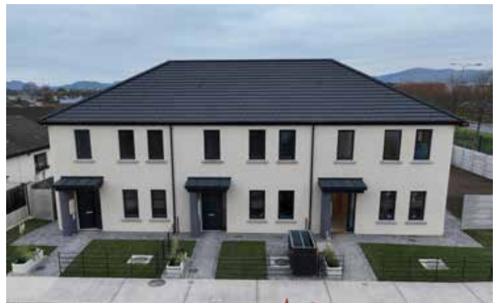
Completed 3D Printed Houses at Grange Close, Dundalk
