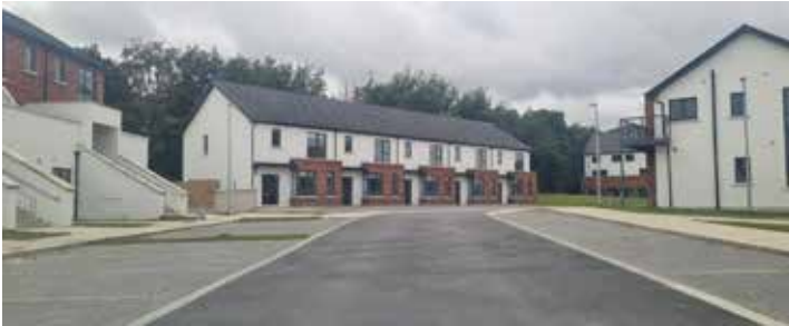
Dublin Road, Dundalk with Respond
