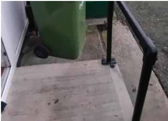
A ramp installed in Dunleer with financial assistance from a HAG.
