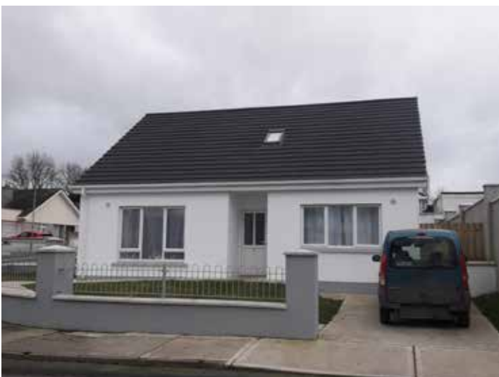
School Lane, Dunleer, completed in 2024 - 1 Unit
