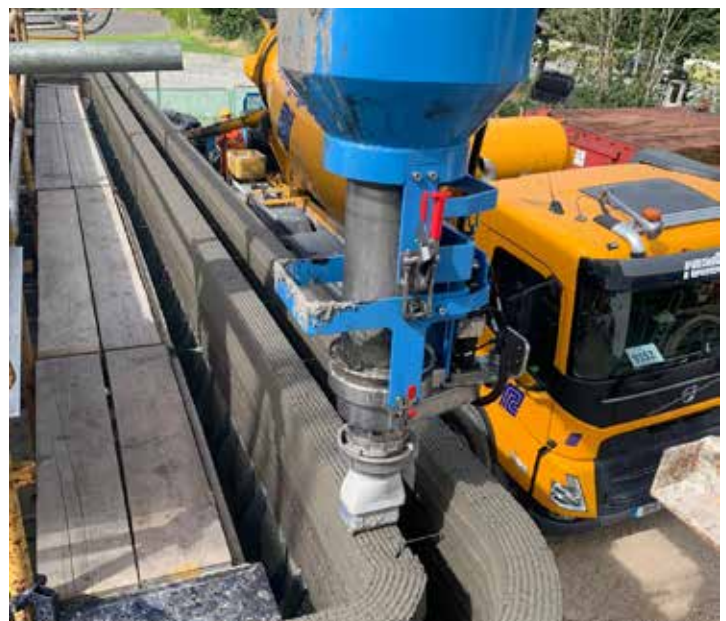
3D Concrete Printer in operation at Grange Close, Dundalk
