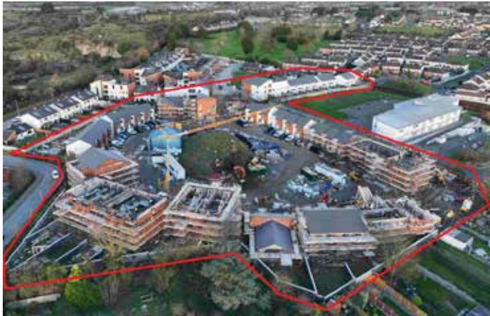
Boice Court, Mell, Drogheda, 72 units under construction
