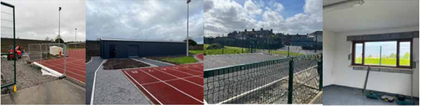
Lourdes Stadium Upgrade Works in Progress During 2024.
