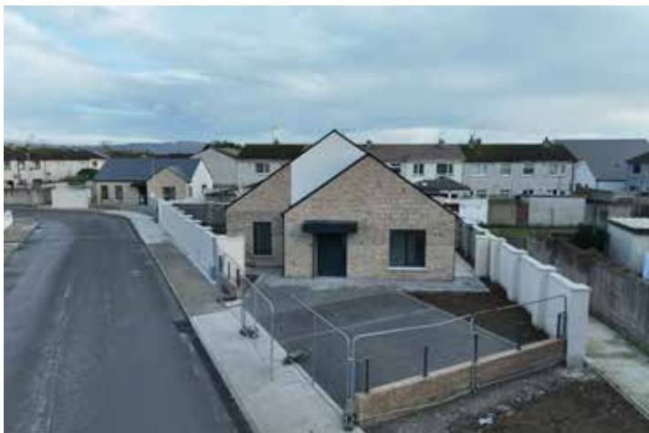
Muirhevnamór, Dundalk, 11 units under construction
