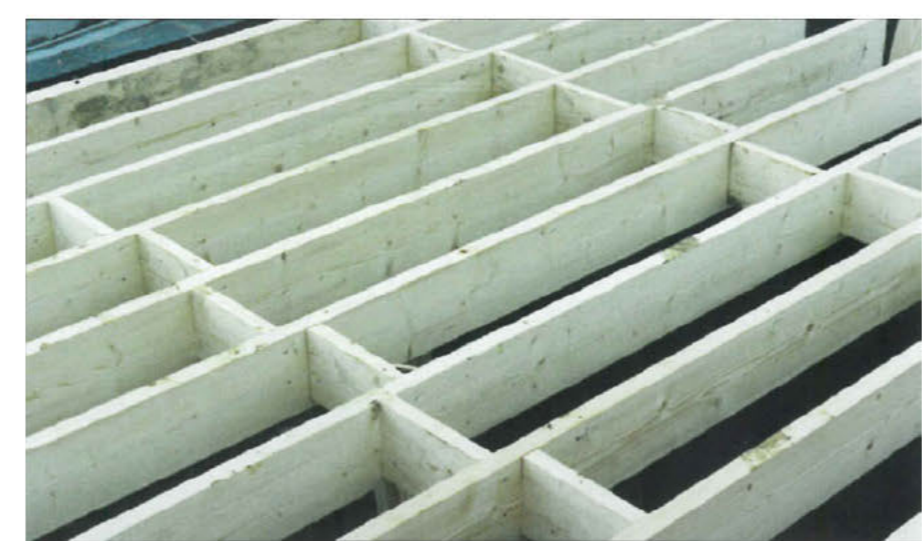
DETAIL 17 Example of solid bridging between joists
